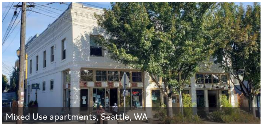
Atrium Apartments, Seattle, WA
