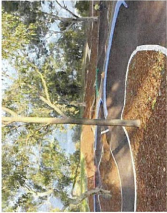
Typical berm treatment with double roller
