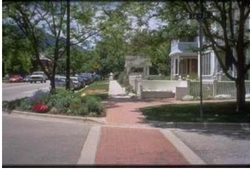
Paving treatments make crosswalks more visible enhancing safety for pedestrians.
